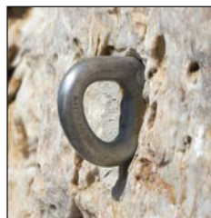
Raumer stainless steel glue-in bolt - good
